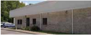
MILESTONE TRAINING CENTER
